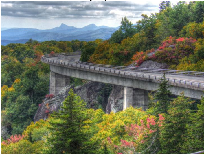
Linn Cove Viaduct at Grandfather Mountain
